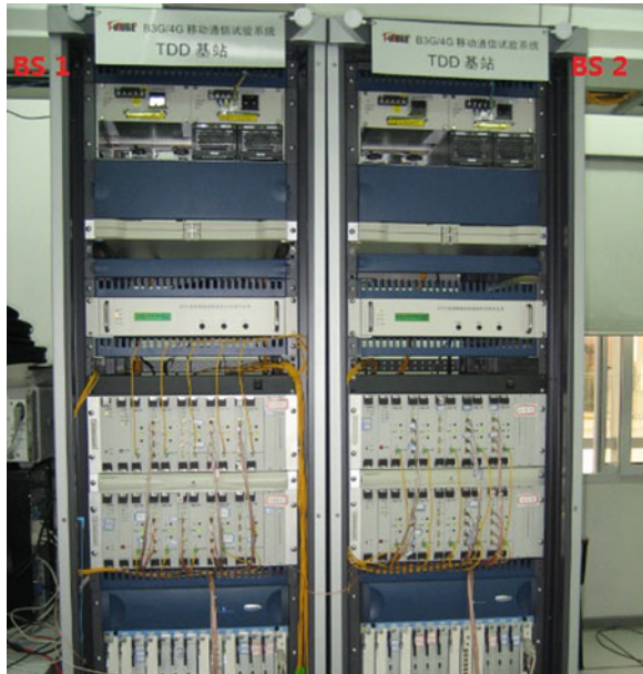
Fig. 5.8 BSs of the FuTURE 4G TDD trial system
